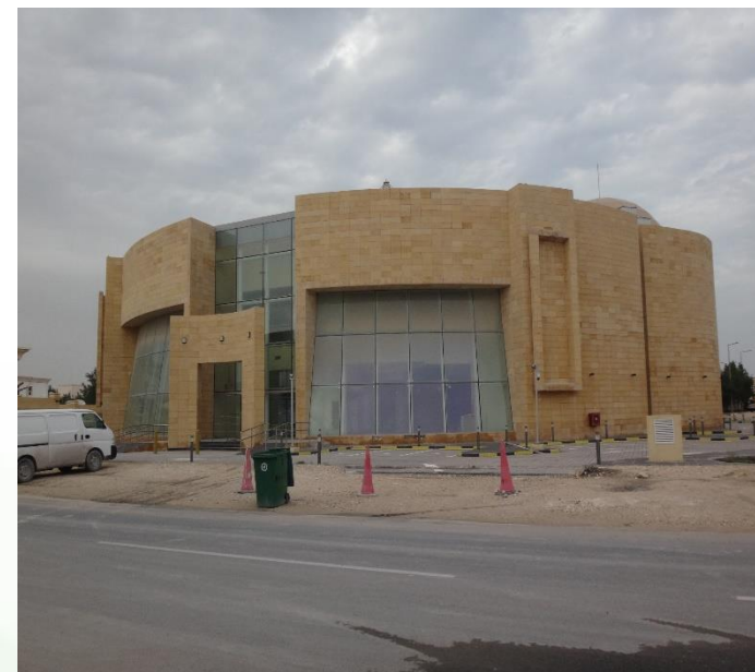
Hypermarket Buildings Doha, Qatar
